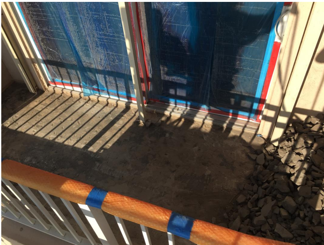
Picture 4: In-progress demolition
