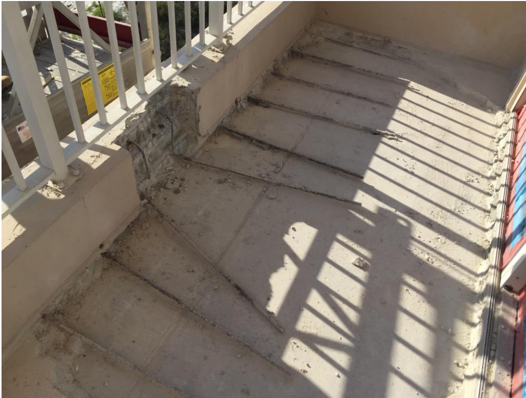
Picture 3: In-progress demolition
