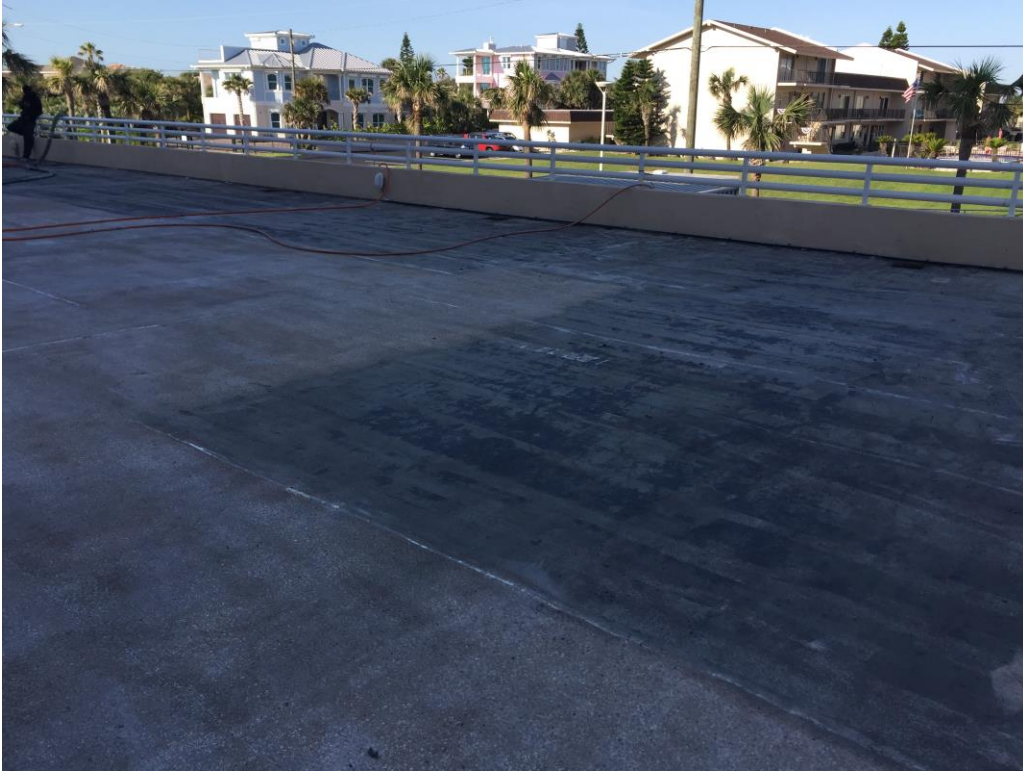
Picture 7: In-progress hydro-blasting
