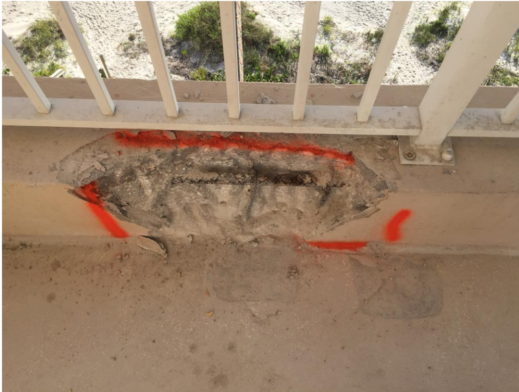
Picture 1: In-progress demolition
