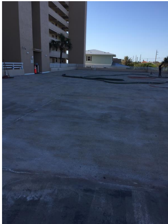
Picture 6: In-progress hydro-blasting
