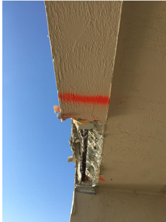
Picture 2: In-progress demolition
