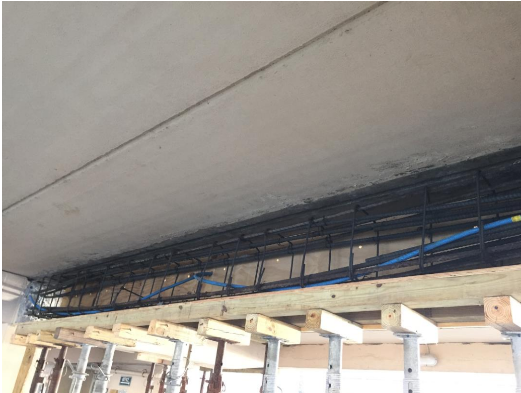
Picture 5: In-progress steel supplementation
